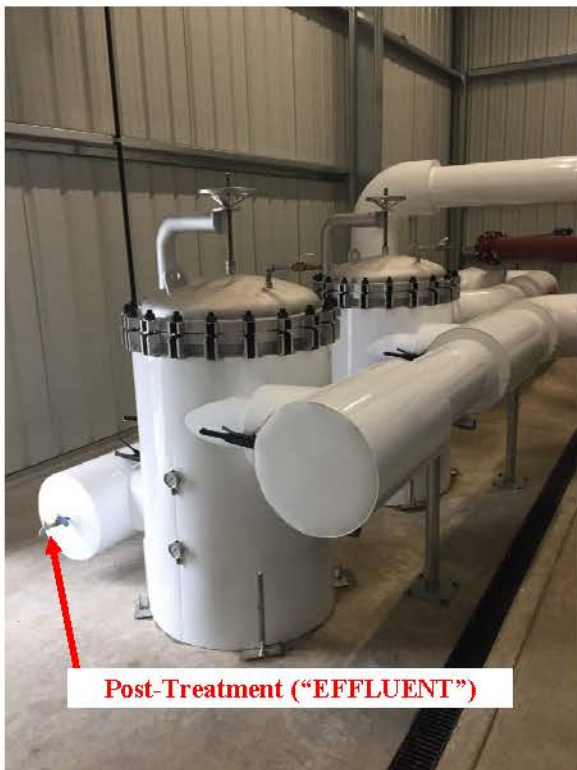
Figure 1—Kroll Well GAC Treatment System Sampling Locations
