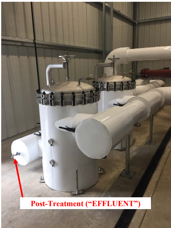
Figure 1—Kroll Well GAC Treatment System Sampling Locations
