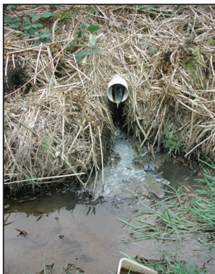
Figure 2: Direct Discharge from a Straight Pipe
