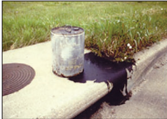
Figure 5: Dumping at a storm drain inlet
