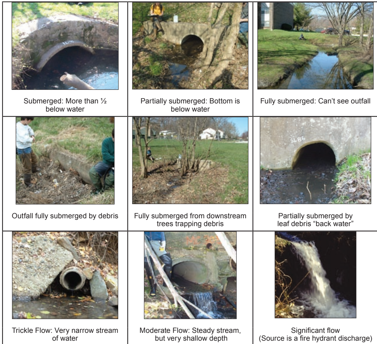
Figure 28: Characterizing Submersion and Flow
