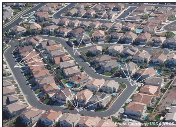
Figure 17: Swimming pools can be a source of illicit discharges.
