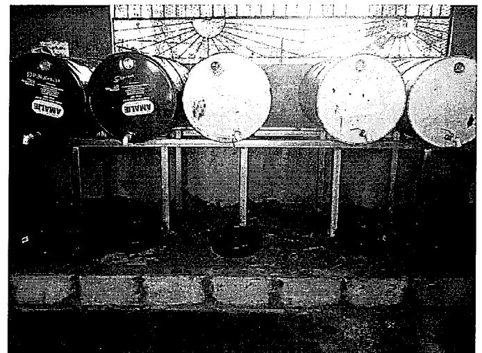
Keeping materials stored indoors and using controls such as drip pans can reduce the risk of a potential stormwater contamination.
