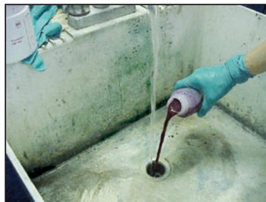
Figure 63: Dye Testing Plumbing (NEIWPCC, 2003)
