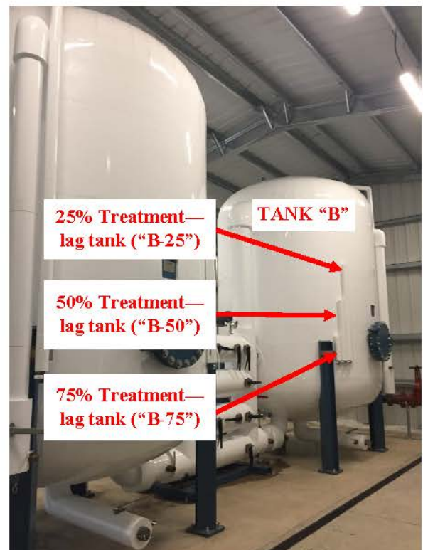
Figure 1—Kroll Well GAC Treatment System Sampling Locations
